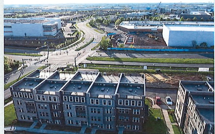
community next to data centers in Ashburn, Virginia.
